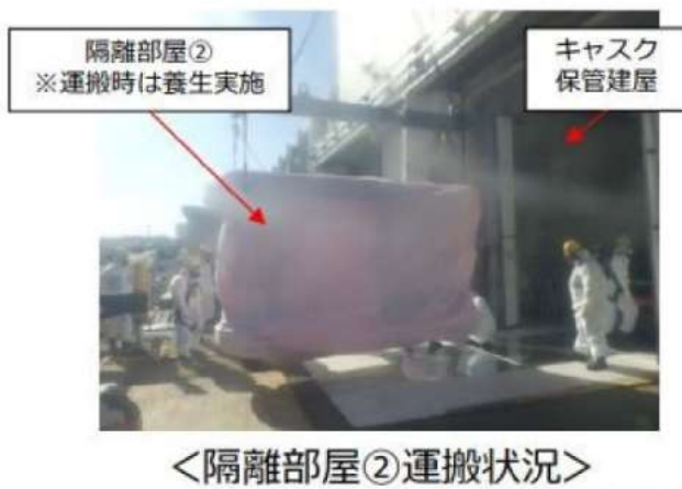
Image: TEPCO. Installation of the hot cell components and a diagram of the same for unit 2.
