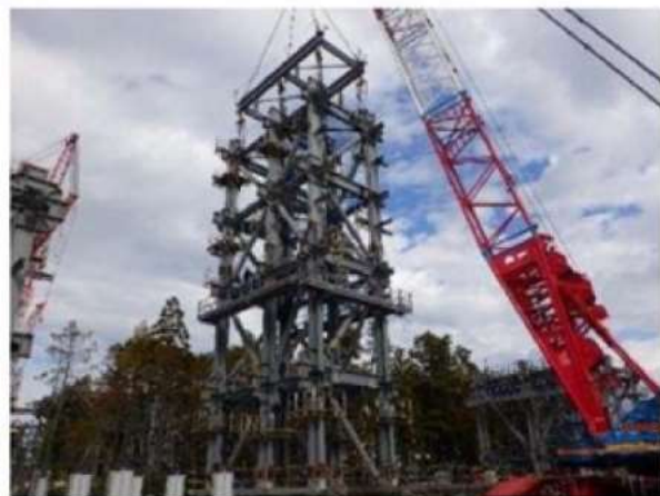
Image: Original Image TEPCO, image enhancement, SimplyInfo.org Unit 2 external defueling building diagram and construction on site.
