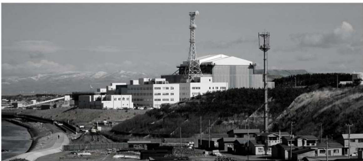
Image: Omha Nuclear Power Plant
